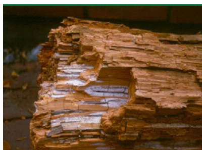
Mine fungus - crack bricks. (Photo: Goritas)
