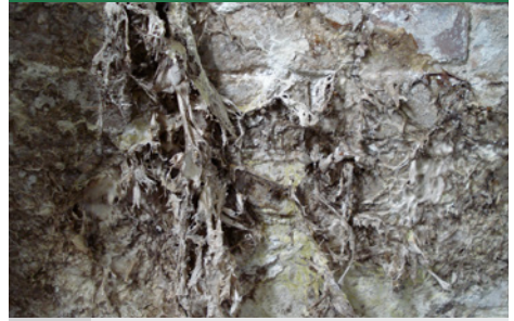
svn 26 Dry rot fungus - older, grey surface mycelium with stringy mycelium. (Photo: Protox)
