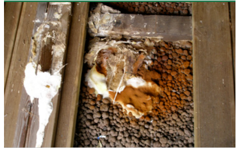
svn 4 Dry rot fungus - fruiting body, cocoa-like spore powder and mycelium on Leca under floor in conservatory. (Photo: Protox/customer photo)
