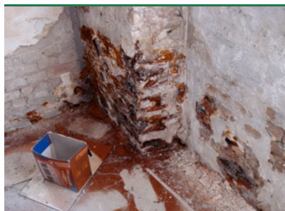
Dry rot fungus - spore powder on floor (from fruiting bodies on wall). (Photo: Protax)
