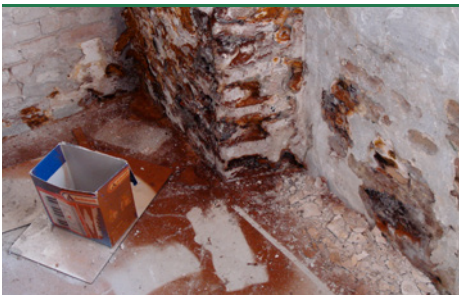
svn 5 Dry rot fungus - reddish-brown spore powder on the floor. (Photo: Protox)
