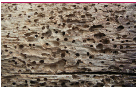
Deathwatch beetle - exit holes in beam. (Photo: Protox)
