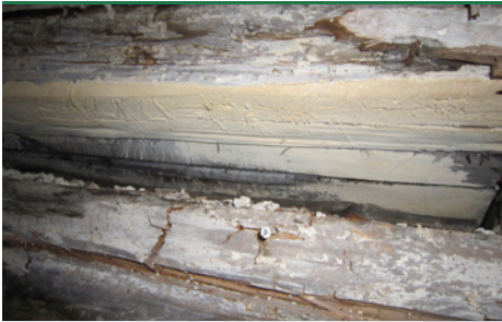
Mine fungus - fruiting bodies and mycelium on decayed wood with crevices. (Photo: Bøgh & Helstrup)
