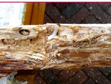
Red-brown Longhorn Beetle in door- post - larva and larval passages with frass. See also page 18. (Photo: Protox)
