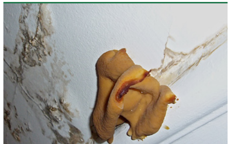
svn 18 Cellar cup fungus - fruiting body on wall by skirting board. (Photo: Bøgh & Helstrup)
